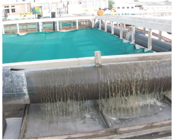
Fig 16: Drum filter before feeding to aeration
