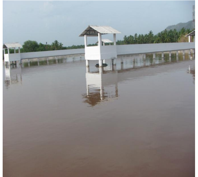
Fig 8 : Primary treated effluent storage tank
