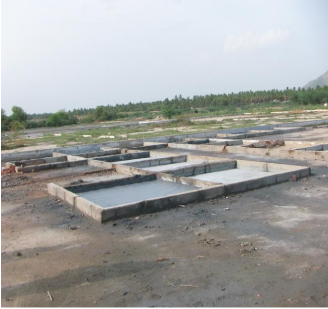
Fig 9: Solar Ponds for drying recovered chromium
