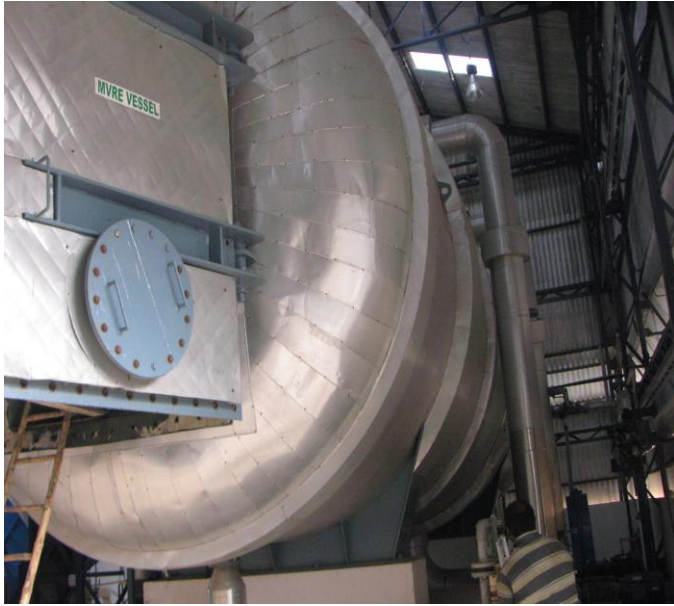
Fig 19: MVRE under maintenance
