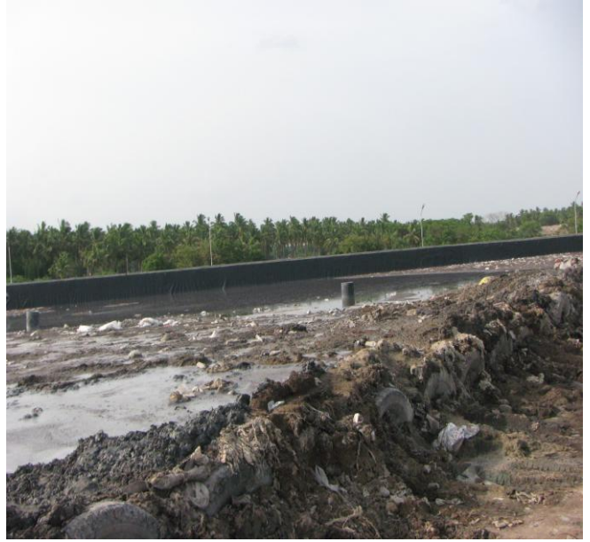
Fig 10: SLF with rain water & leachate
