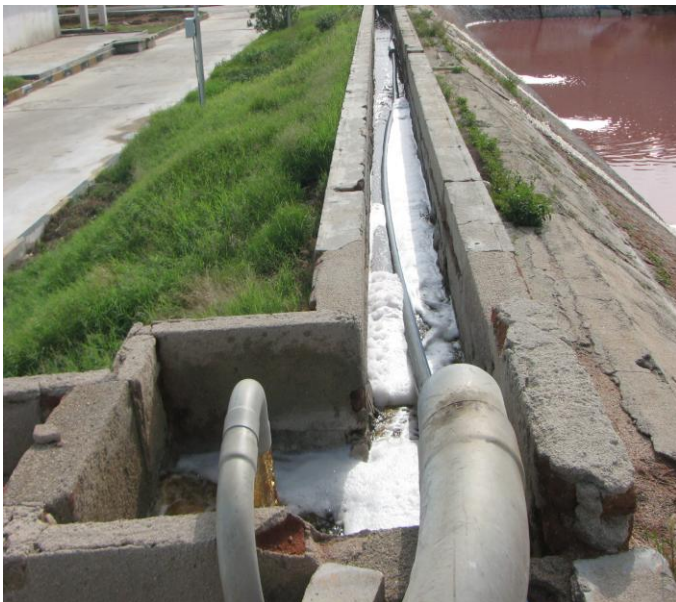
Fig 7: R.O. Reject Collection
