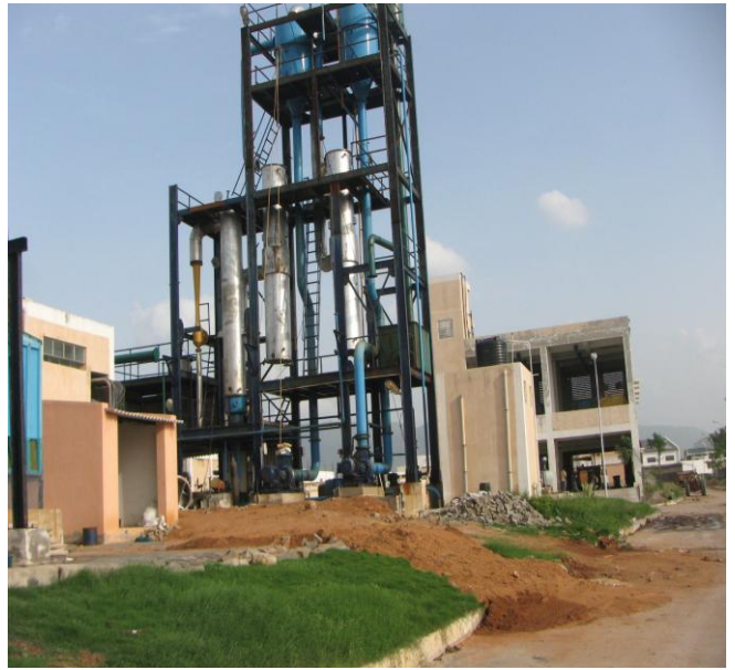
Fig 20: Multi Effective Evaporator under repair
