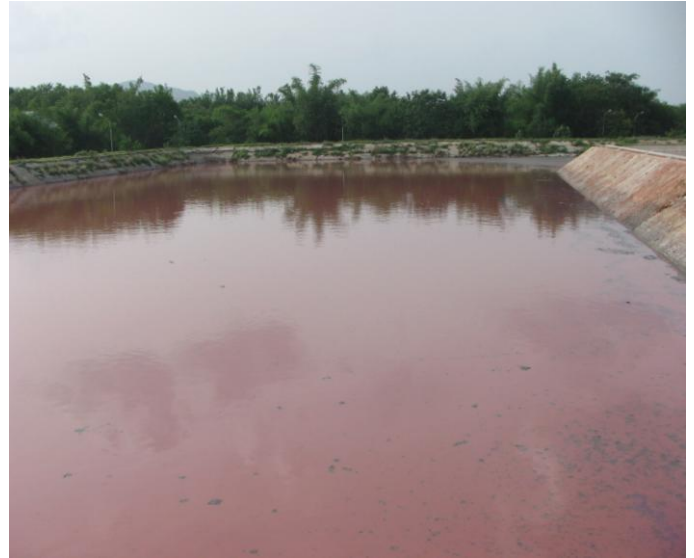
Fig 6: R.O Reject Storage Tank
