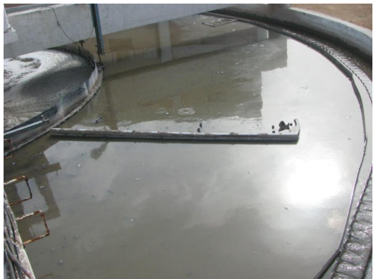
Fig 4: Secondary Clarifier
