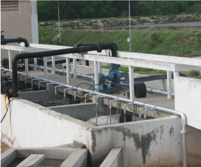
Fig 5: Sieve filtration system
