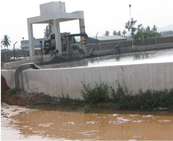
Fig 1: Effluent receiving tank
