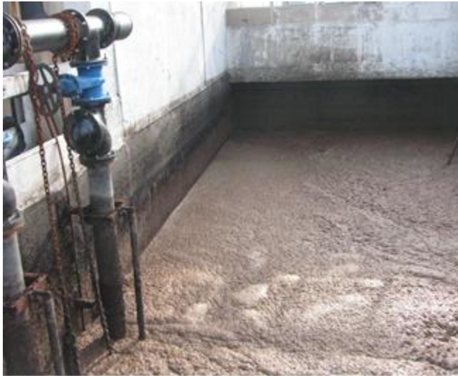
Fig 13: Aeration Tank
